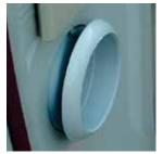
Mark out and cut a 70mm hole for the filler point
