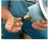
Install the Brass Filler head into the bracket using the 4 screws and bracket provided
